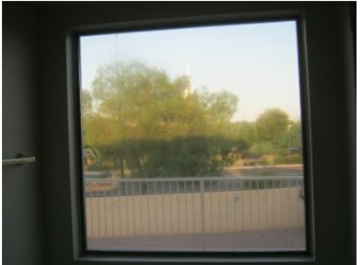
Broken seal(master bath).
