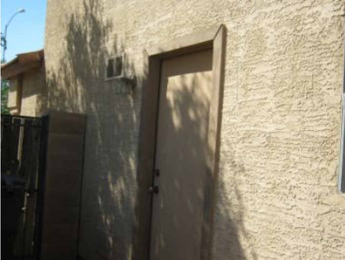
Garage side door exterior trim and door jam are deteriorated. We recommend repair.
