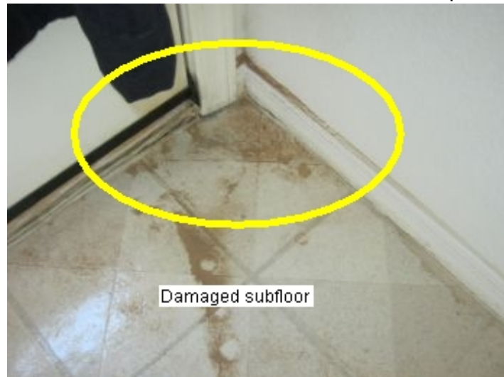
The master bedroom balcony door jam is deteriorated and we also noted damaged to the sub-floor at the inside of the door. We recommend further evaluation and remedy by a competent contractor.
