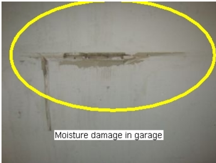
Moisture damage in garage.
